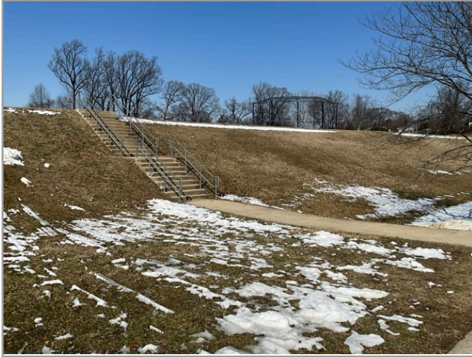
ACCESSIBLE ROUTE TO PLAYGROUND
