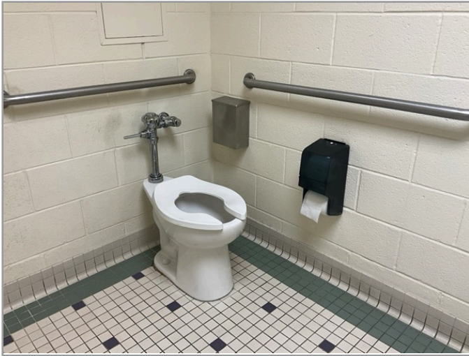
TOILET STALL OVERVIEW
