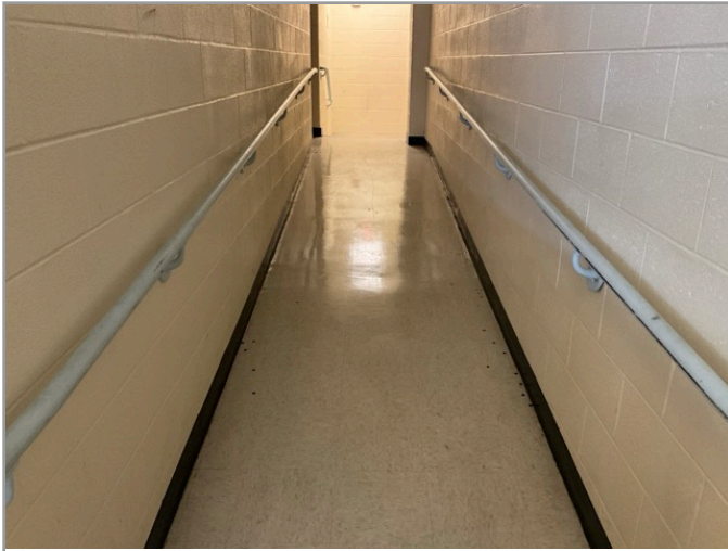
ACCESSIBLE INTERIOR RAMP
